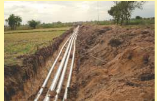
Installation of Supreme pipeline in the field
