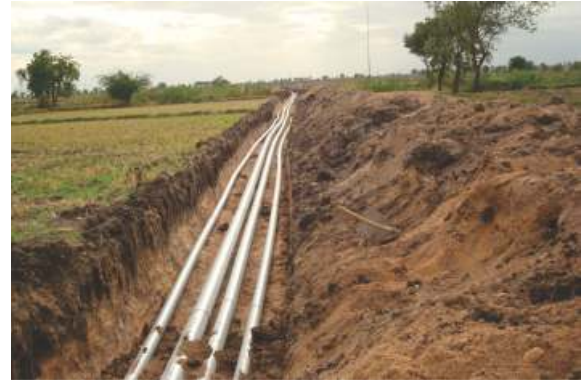
Installation of Supreme pipeline in the field
