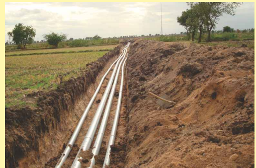
Installation of Supreme pipeline in the field
