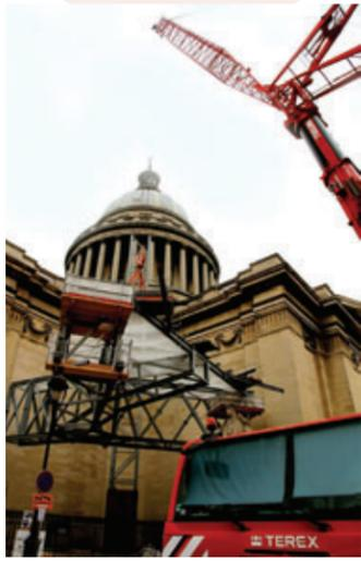
With the passing of the years, the pressure on its arches, water seepage caused by leaky joints and the corrosion of swelling metal components which have cracked open surrounding stone has compromised the stability of the structure. That is why the Centre des Monuments Nationaux, the main caretaker for the national monument system, has now undertaken a massive restoration project. The first phase of this restoration work will last until 2015, starting with the upper part of the structure at
