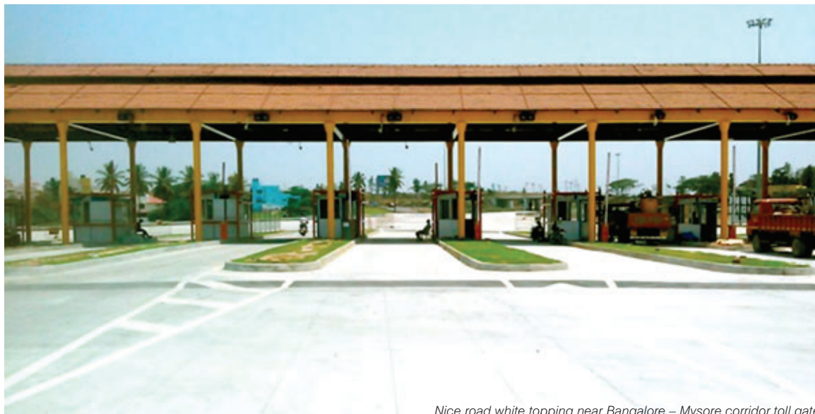
Nice road white topping near Bangalore - Mysore corridor toll gate
