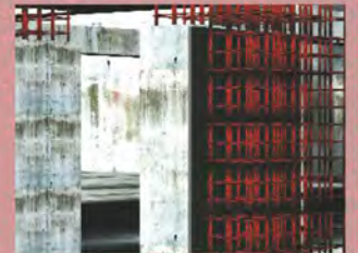
DURAboardHD100 used in expansion joints in columns
