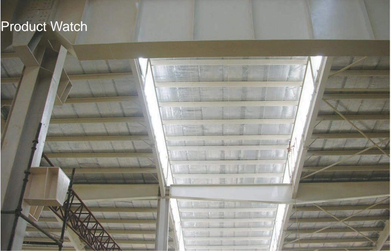
with its multiple layers of aluminum and enclosed air space (INSUreflector), is positioned in a building cavity (stud wall, furred-out masonry wall, floor joist, ceiling joist, etc.) to divide the larger cavity (3/4" furring, 2" x 4", 2" x 6", etc.) into smaller air spaces. These smaller trapped air spaces reduce convective heat flow.
