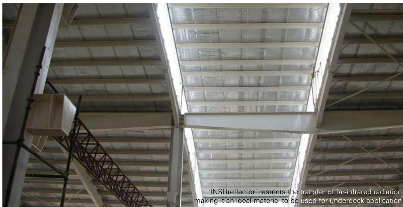
'INSUreflector' restricts the transfer of far-infrared radiation making it an ideal material to be used for underdeck application
