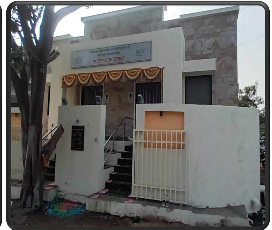
Public Sanitation Facility at Jalgaon (Maharashtra)
