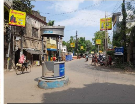
Traffic Signal at Bankura, West Bengal
